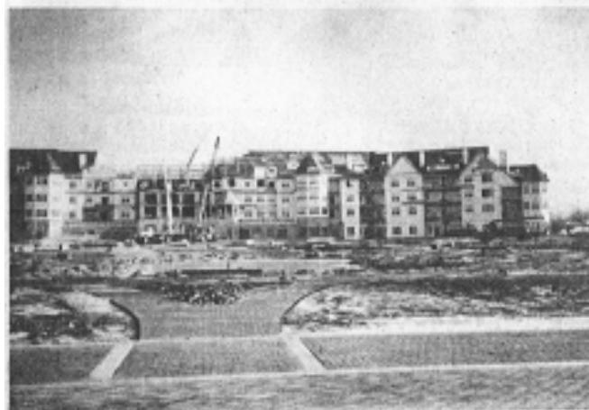
THE OSTHOFF BUILDING — View from lakeside walk shows how both ends of the building have been enclosed, while construction continues on the center section.
